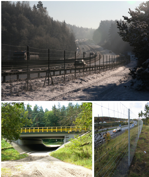
Figure 2. General view of the fenced section of the Tri-City Bypass (top) and of one of the underpasses with visible fence in sides (bottom left), fence with visible differentiated, height-dependent mesh size (bottom right). All photos DJ.
